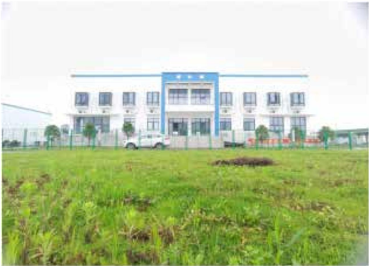
Figure 15 Greening in the booster station
