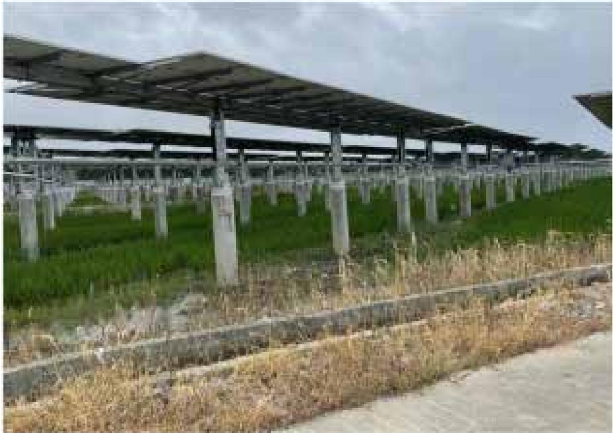
Figure 5 Recultivation of land under photovoltaic panels
