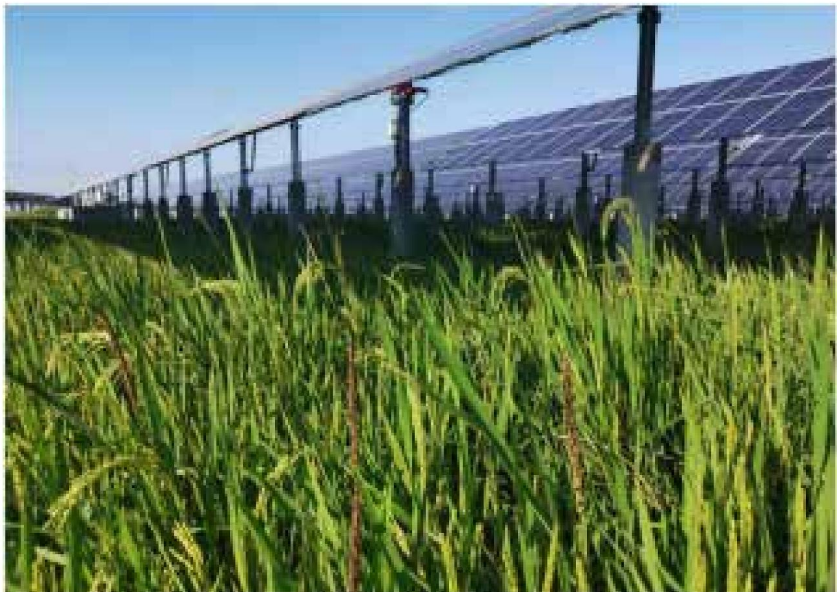
Figure 6 Recultivation of land under photovoltaic panels
