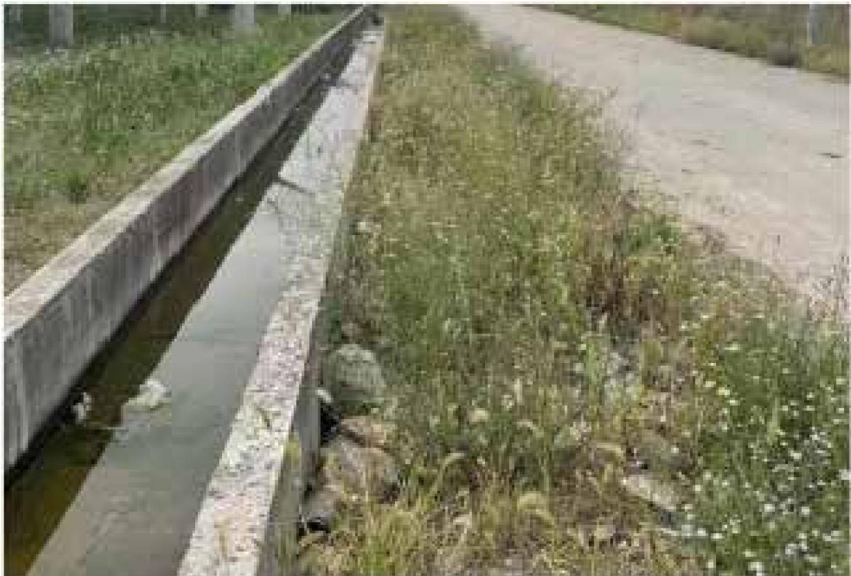
Figure 12 Drainage ditches on both sides of the road
