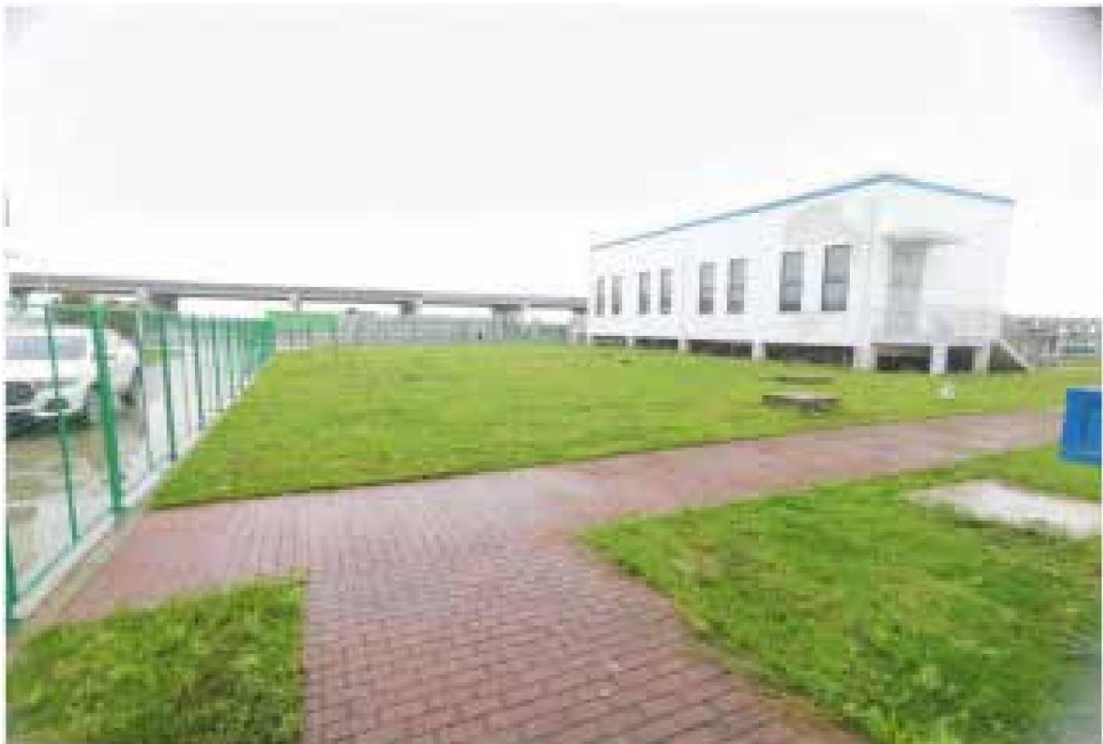
Figure 16 Greening in the booster station
