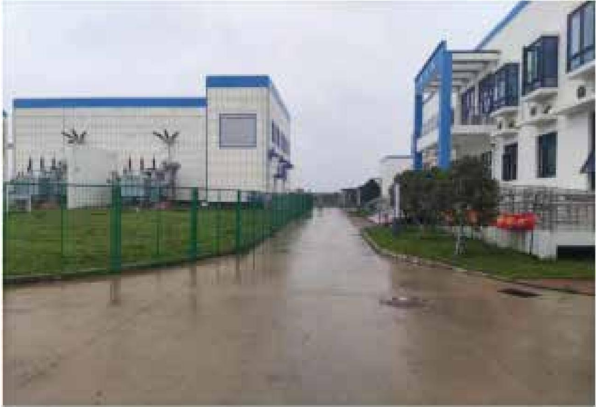
Figure 17 Greening in the booster station
