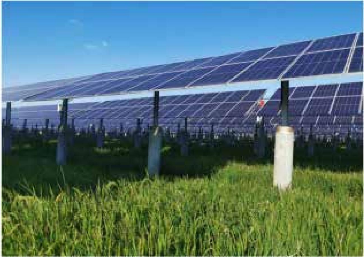
Figure 7 Recultivation of land under photovoltaic panels
