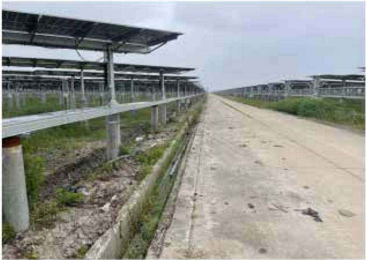
Figure 13 Drainage ditches on both sides of the road
