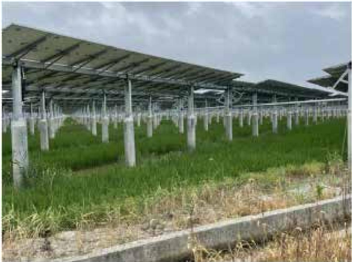
Figure 4 Reclamation of land under photovoltaic panels
